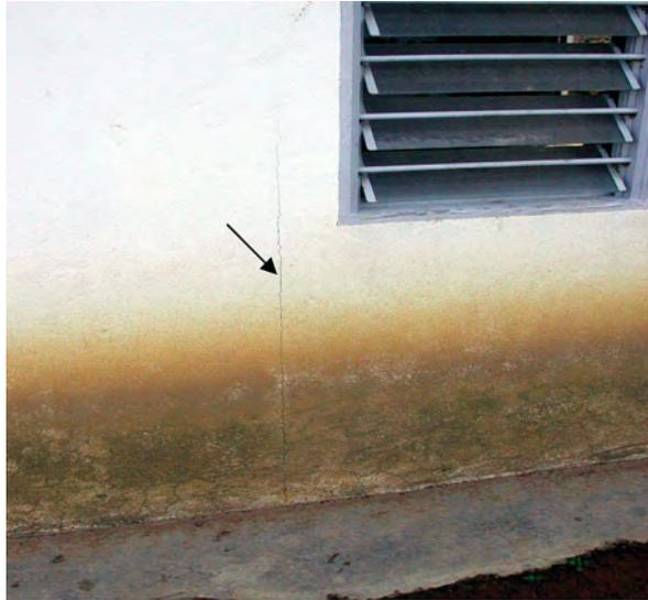
**Figure 2:** Hairline cracks on the wall at a house; the crack on the wall goes all the way through the house. Location: Kampong Chemperoh.
