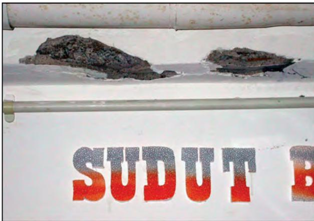
**Figure 3:** Chunks of cements had fell off the ceiling of a ground floor laboratory. Location: Sek. Men. Bukit Tinggi.
