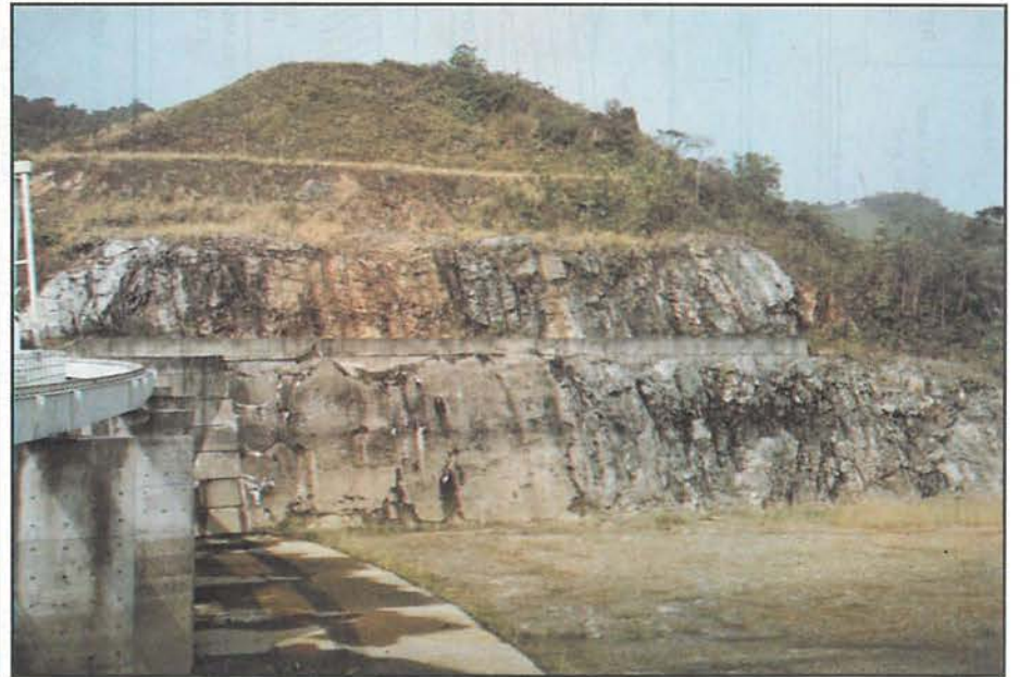
Figure 9. Gabbro sills (on right) intrusive into Lupar Formation, west abutment, Main Dam.
