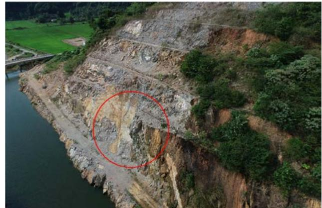
Figure 6: Site condition on possibility of failure through planar sliding.
