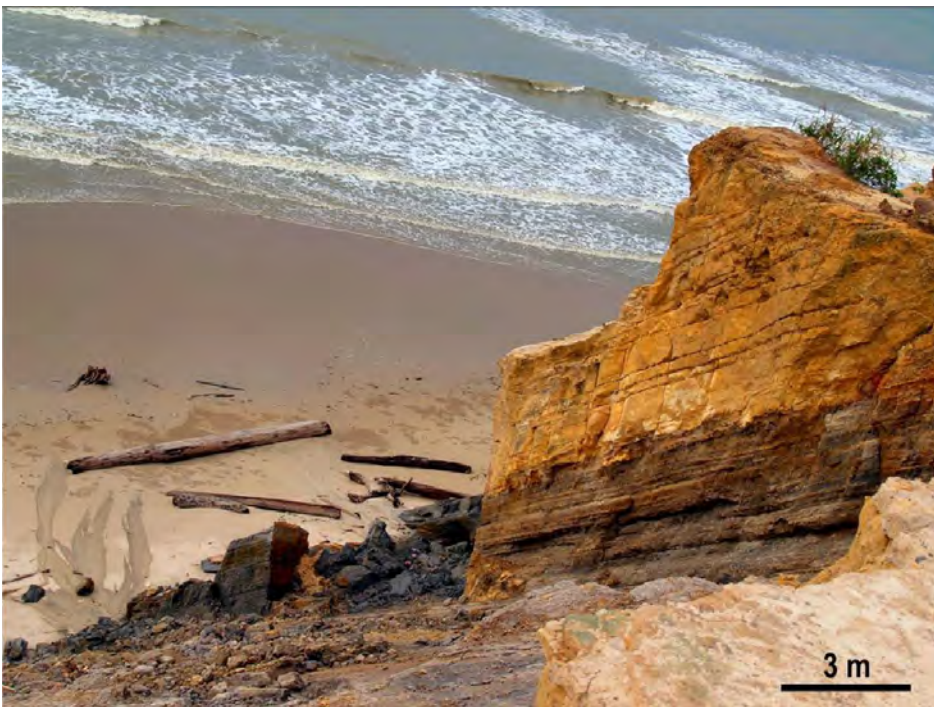
Figure 4: The seaward-dipping clay sections form ideal gliding surfaces, and particularly after strong rainfalls the rock face becomes unstable and collapses.
