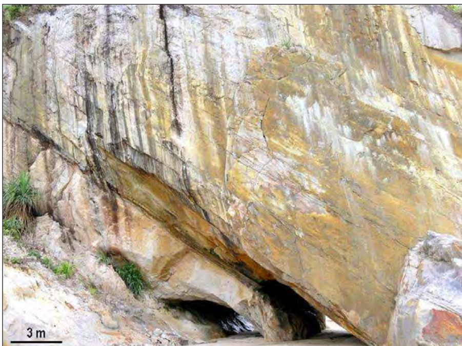
Figure 13: In 2010, longshore currents and bio-erosion started to scour the promontory, and created caves which grew in size over time.
