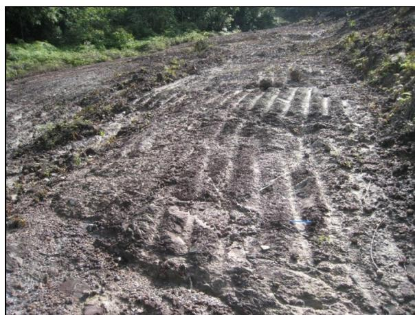
Figure 4: Teeth marks (10 cm width) of scrapers on slightly weathered quartzite.
