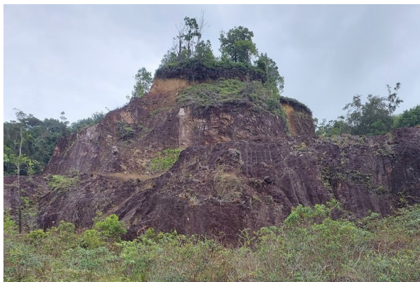
Figure 2: Excavation in Sungai Perlis Beds on west side of Bukit Teluk Batu.
