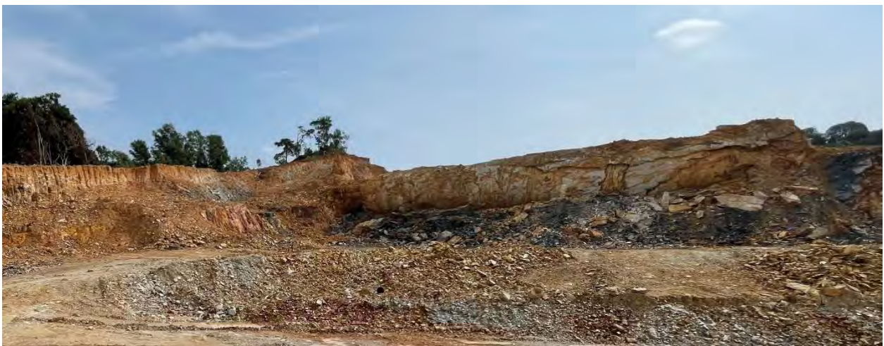
Figure 4: The northeast wall of the quarry and black shale.
