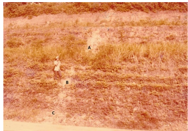
Figure 3: View of slope cut with sampling locations.
