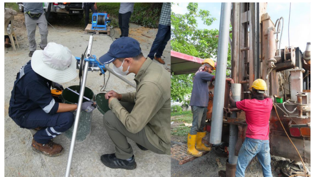
Figure 7: Image on the left shows the downhole geophysical logging conducted before the PVC installation, as shown on the right.
