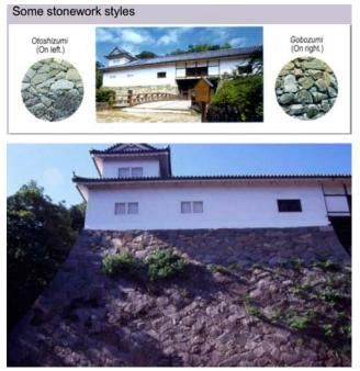
**Figure 7:** Stonework of Hikone Castle. Two-storied turret at the gates, which has been repaired many times, especially in 1854. The stone wall of right hand side was made in the original Gobozumi style of stone work. The left side was made by the later Otoshizumi style, because it was destroyed by the earthquake and re-built.
