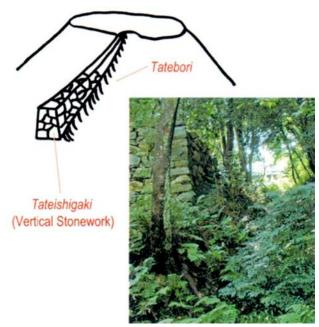
**Figure 8:** Vertical stoneworks, "Tate-ishigaki" in Japanese. "Tate" stands for vertical, and "ishigaki" is stonewall. Vertical stoneworks run from the top to the bottom of a hill to prevent an enemy attack. The top of the stonework is surrounded by a wall with tiles on top.
