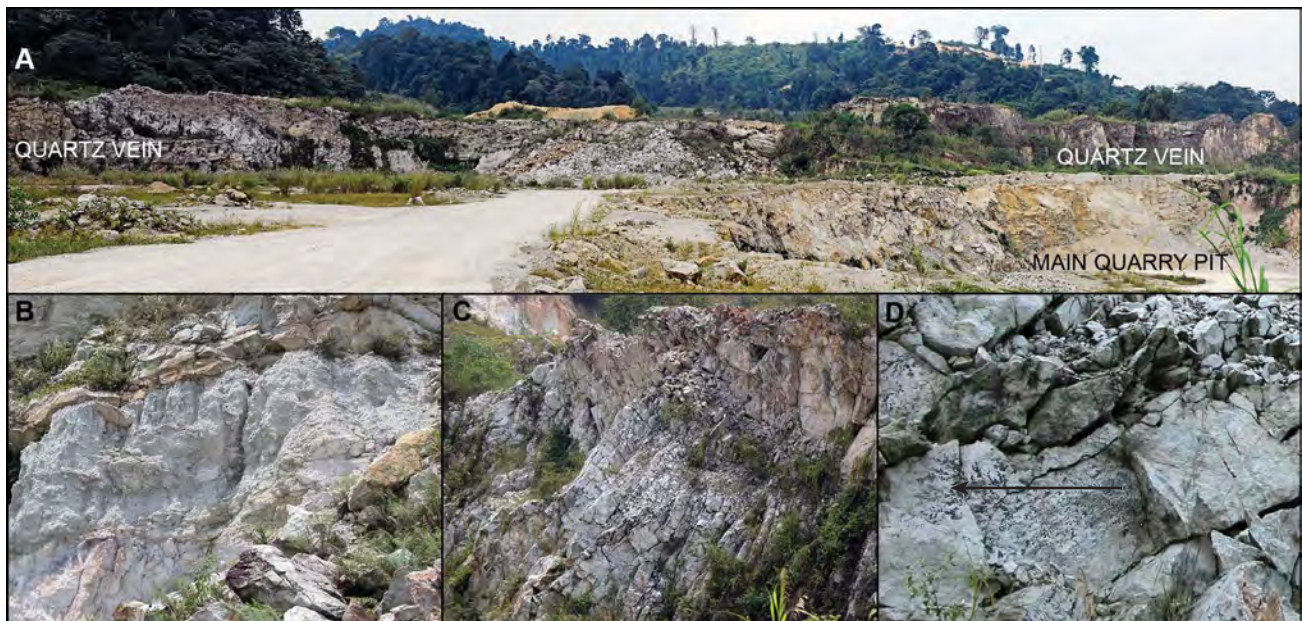
Figure 2: A) Photograph of the quartz vein exposure along the northern face of the main quarry pit. B) A zone of fault breccia occurring along southwestern boundary between the quartz vein and granite. C) The quartz vein is well jointed and the most prominent joint set is subparallel to the vein and fault. D) Manganese dendrites with subhorizontal growth axis (arrow).
