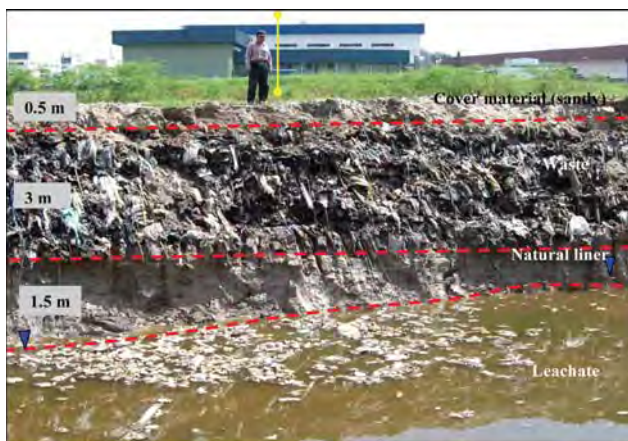
Figure 6: Photograph of the excavated part of Bukit Kemuning Landfill.
