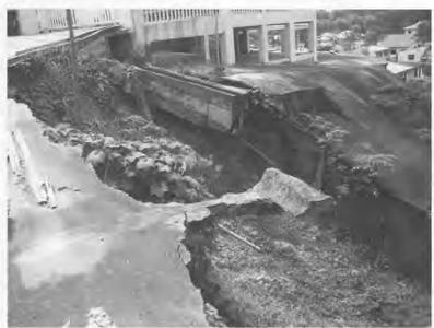
Figure 9. Foundation problems associated with the Crocker Formation (Location: Bukit Padang)
