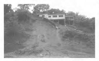
Figure 4. Slope failure at Bundusan road, Luyang
