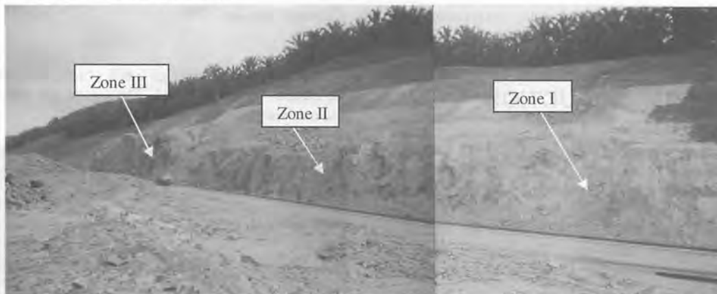
Plate 2: Overall view of the right hand side cut rock slope
