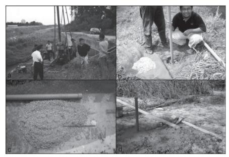
**Figure 4.** Field investigation scenes. a) Standpipe installation. b) Gravel packing material and PVC standpipe. c) Installing of the PVC standpipe. d) Completed standpipe.
