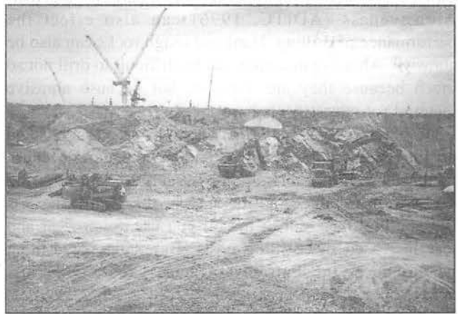
Figure 6. Closer view of the Putrajaya gneiss outcrop.
