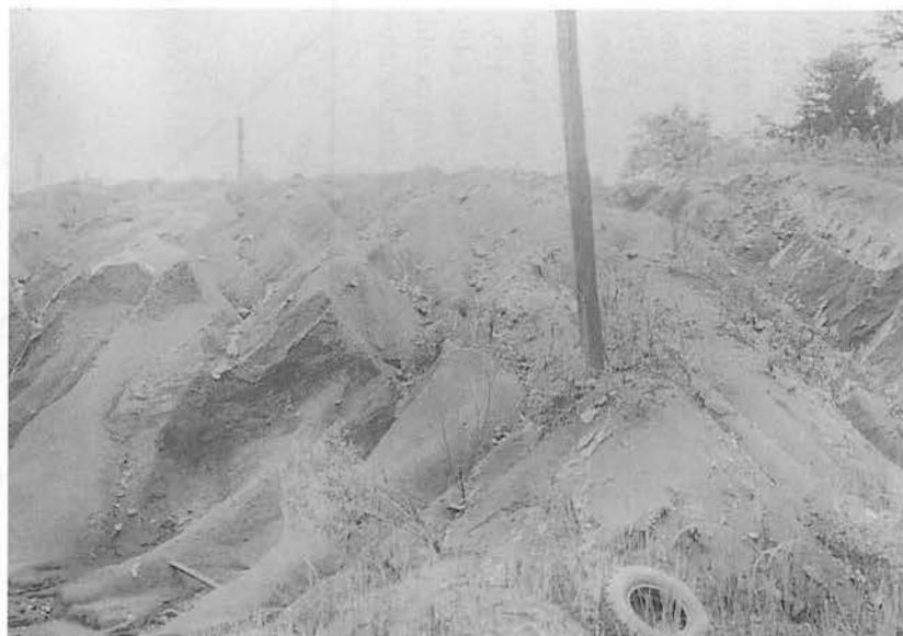
Figure 6. Intensely sheared thick mudstone beds with calcite veins of the Labang Formation. The shearing (dipping to the left) trending NE-SW is probably associated with the Lonod Fault. Locality near Sabah Forest Development Camp, about 40 km southeast of Sapulut.
