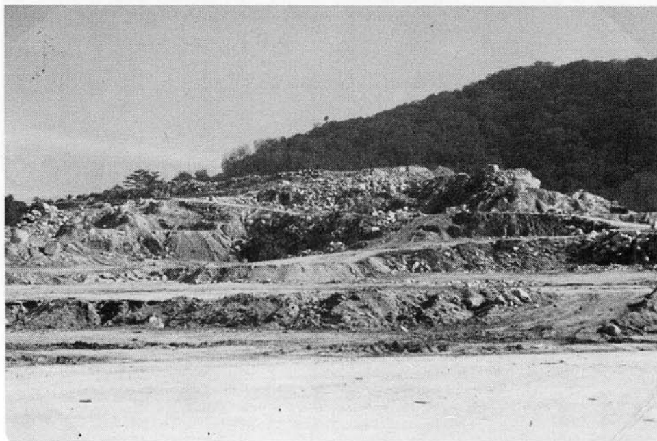
Plate 4. Excavated site showing highly irregular bedrock topography typical in tropical terrain. No well-defined plane interface exists between the overburden and the sound bedrock. (Taman Tun Dr. Ismail, Kuala Lumpur).
