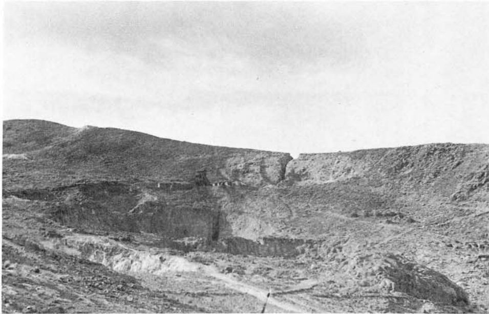
Plate 1. Surface subsidence at Llallagua due to underground mining activities.
