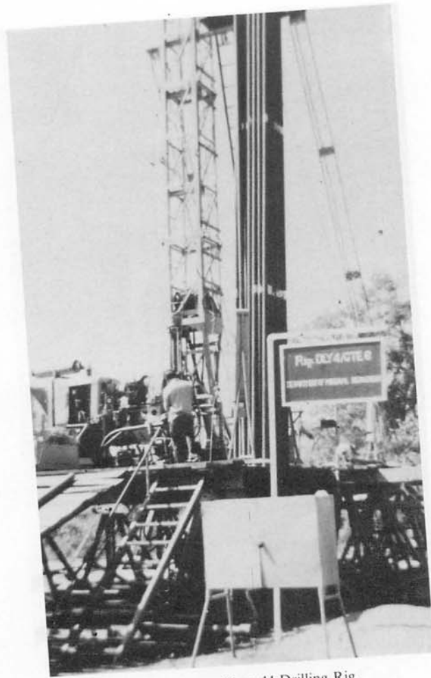
Plate 1. Long Year 44 Drilling Rig.
