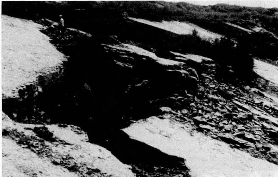
Fig. 7. The planar slides on the southeastern slope. The sliding blocks move along the bedding planes which dip gently into the mine pit.
