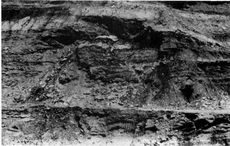
Fig. 5. The continuation of the 1980 wedge failure (Figure 4) as observed in March 1981.
