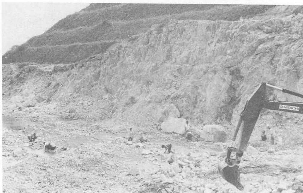
Plate 1: Eastern half of the roadcutting. Foreground shows a number of tin-fossickers at work. Note about 30 m thick of residual soil has been removed (background).
