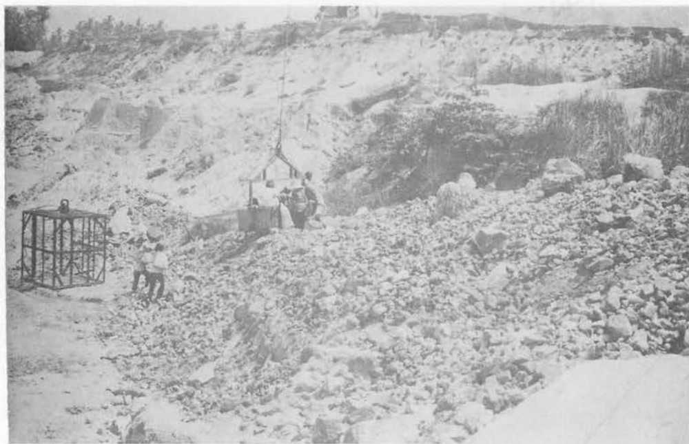
Plate 3 Foreground shows the mine dump with the rock boulders. Immediate background shows a group of cassiterite scavengers running to search for cassiterite from a new of rock boulders just lifted up by the crane from the mine hole. Steel cage on the left is used to lower and lift up workers.
