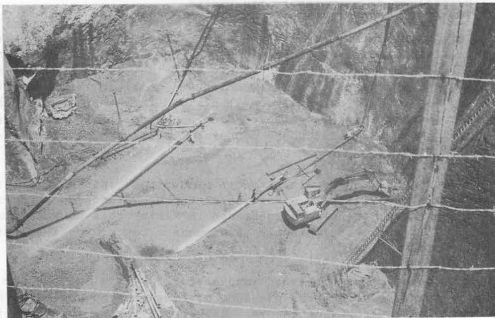
Plate 1 Looking down the mine hole from the top. The hydraulic excavator and the monitor pumps are in operation. Note the smoothness of the side wall. The first stage vertical pump is on the left.
