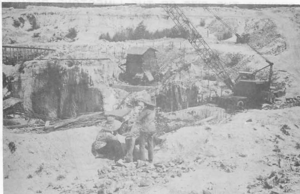
Plate 2 Top of the mine, looking west. Part of the top of the pothole is visible. Hut with second stage vertical pump and lift crane are in the immediate background
