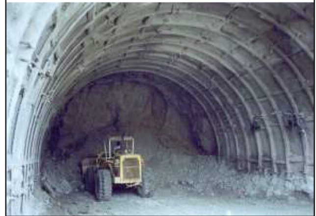
Figure 21a, 21b: Highly fractured granite and steel sets support, diversion tunnel, Sg. Selangor dam.
