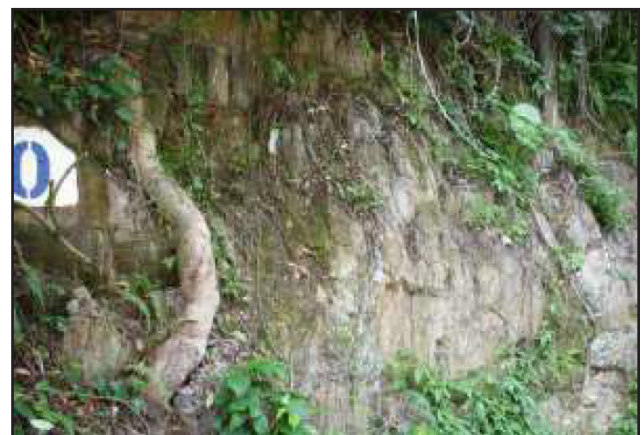
Figure 20: Root wedging along joints in quartzite of the Kenny Hill Formation, Kuala Lumpur.
