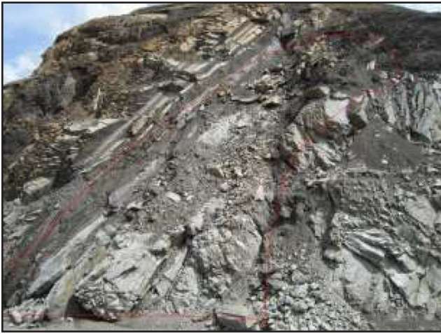
Figure 18: Failure in black carbonaceous shale due to ravelling and erosion, Belaga Formation, Sarawak.
