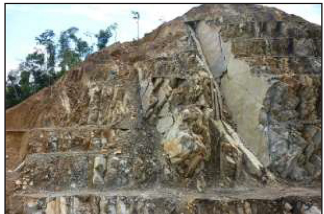
Figure 17: Major plane failures along bedding planes in sandstone of the Belaga Formation, Sarawak.
