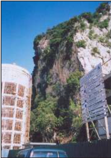
Figure 8: Water tank at Batu Caves limestone cliff, Kuala Lumpur.
