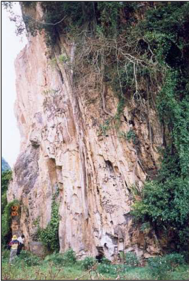
Figure 7: Sub-vertical bedding planes giving rise to rockfall, Tambun, Ipoh.
