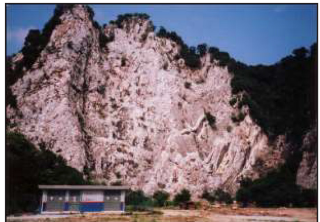
Figure 10: Limestone cliff adjacent to proposed Condominium “B”, Batu Caves, Kuala Lumpur. The cliff face is an ex-quarry face which has been blasted to < 90^\circ . Bedding planes can be seen on the lower right corner of the quarry face.
