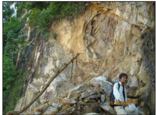
Figure 19b: Toppling failure due to sub-vertical joints in sandstone, Bakun Dam, Sarawak.
