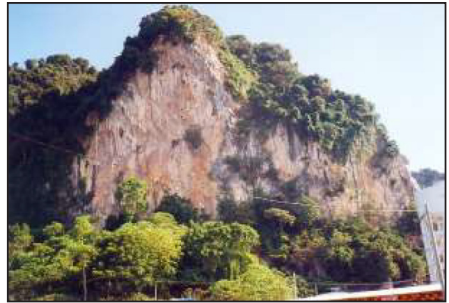
Figure 9: Overhanging limestone cliff adjacent to proposed condominium “A”, Batu Caves, Kuala Lumpur. Lower half of cliff has fallen previously, producing rockfall debris at the base of the cliff.
