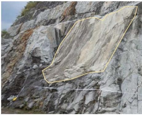
**Figure 1:** An example of planar failure scar at Slope L3 in Rawang. The scar was estimated to be 2 m wide and 3 m high with smooth releasing planes at the sides.
