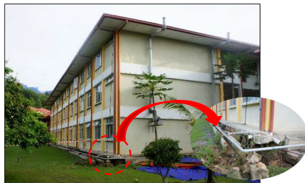
Figure 1: On site slope condition, red circle mark as Point A.
