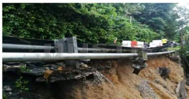
The landslide along Jalan Bayan Lepas towards Balik Pulau, Penang on Thursday, 19 th October 2018. Source The Star Online website
