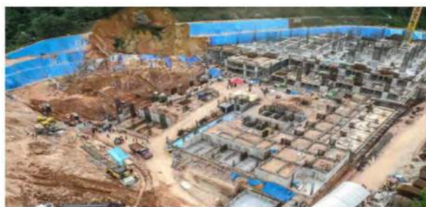
Tanjung Bungah Landslide, Penang, Malaysia on Saturday, 21 st October 2017. Source: Malaymail website
