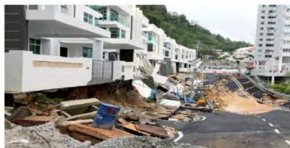
The landslide along Jalan Persiaran Tanjung Bungah, George Town on Saturday 4 th November 2017. Source New Straits Times website
