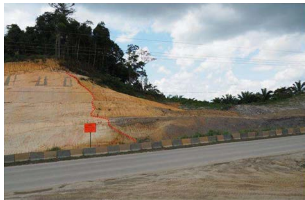
Figure 5b: Close-up of Figure 5a showing faulting (dashed red line to the right of warning panel).
