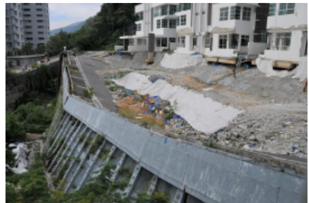
Figure 3: The front view of the collapsed retaining wall and road structures at Beverly Hills in Tanjung Bungah, Penang.
