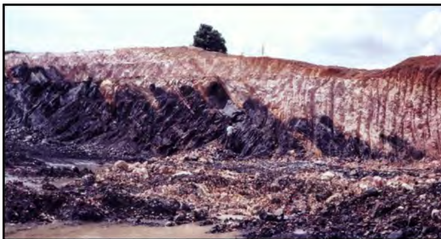
Plate 1: View of shales and sandstones during excavation works.
