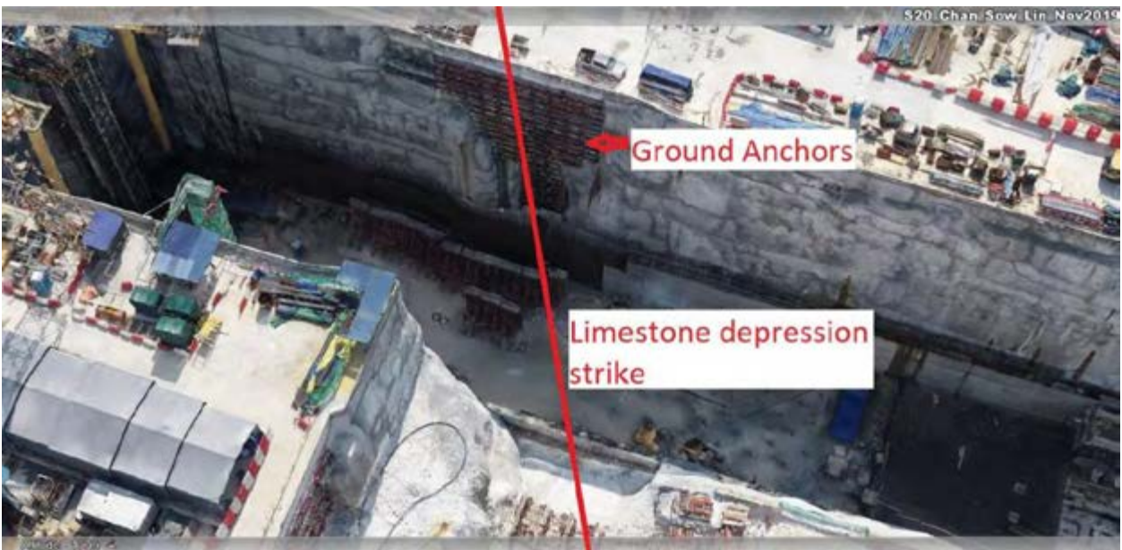
Aerial view of Chan Sow Lin station showing deep depression in limestone and ground anchors.
