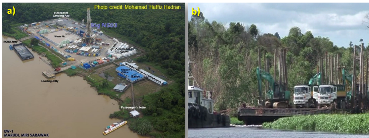
Figure 4: a) Drill site location of exploration well Engkabang West, near the bank of upstream Baram River, Marudi (photo credit: Mohamad Haffiz Hadran) where, b) crew changes and moving of rig, trucks, heavy machineries, cabins and logging tools were done by river transportation, which played a critical role in the drilling operations.
