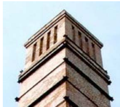
Top and iron bands on The Chimney.
