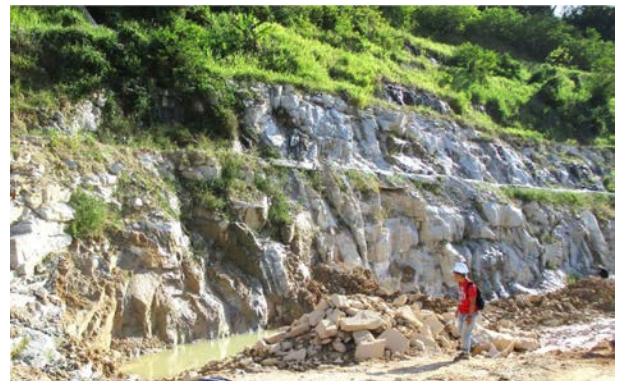
Figure 4: Overview of weathering profile of grade II – III at circle A area of Figure 2.
