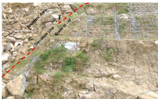
Figure 6: Overview of weathering profile of grade III – IV at circle B area of Figure 2.
